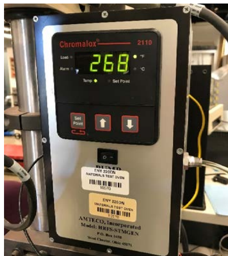
Figure 13: AMTECO steam generation system
