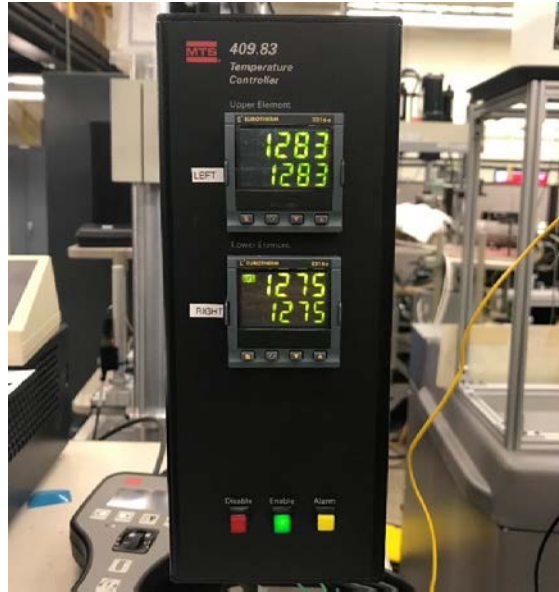
Figure 10: MTS Temperature Controllers
